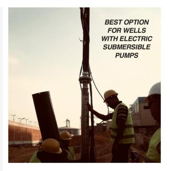
Suitable for pump settings up to 120 metres, Wellman 120 is used in applications such as domestic, light industrial, remote areas and well test pumping.
