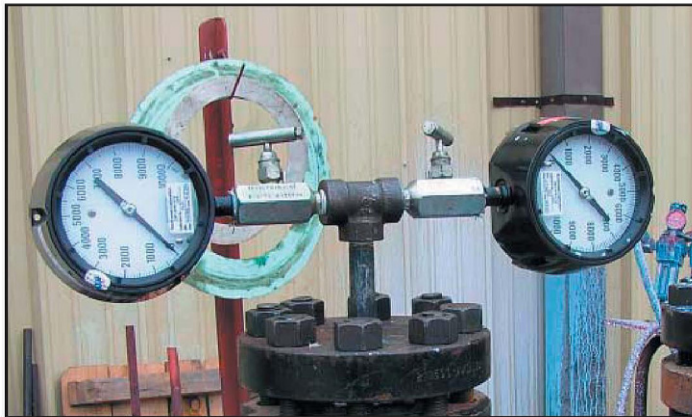
←← Pressure Gauges during testing
