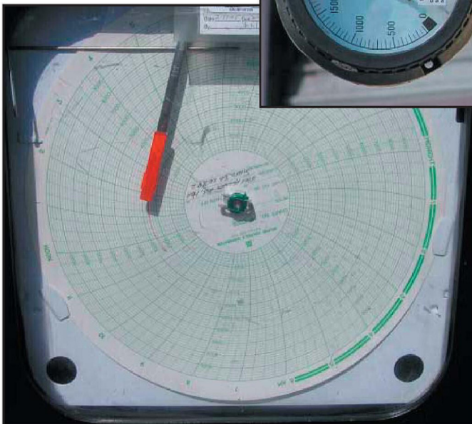
← Flow Meter tracking pressure during hydro testing.
